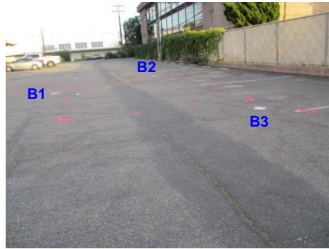
Boring locations B1, B2, and B3.
