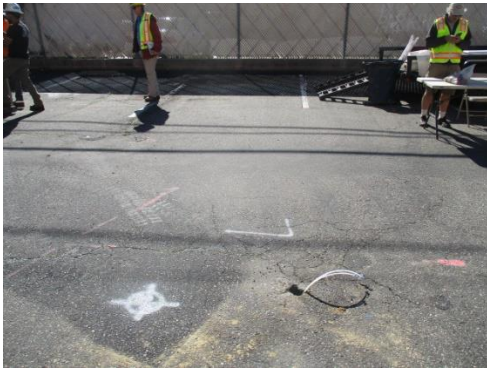
Boring B1 looking south.
