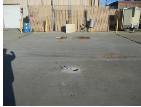
Boring B4 looking east.
