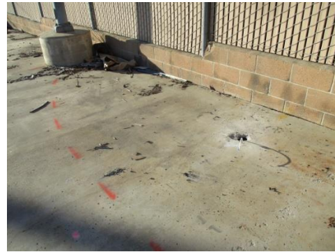
Boring B6 looking northwest.
