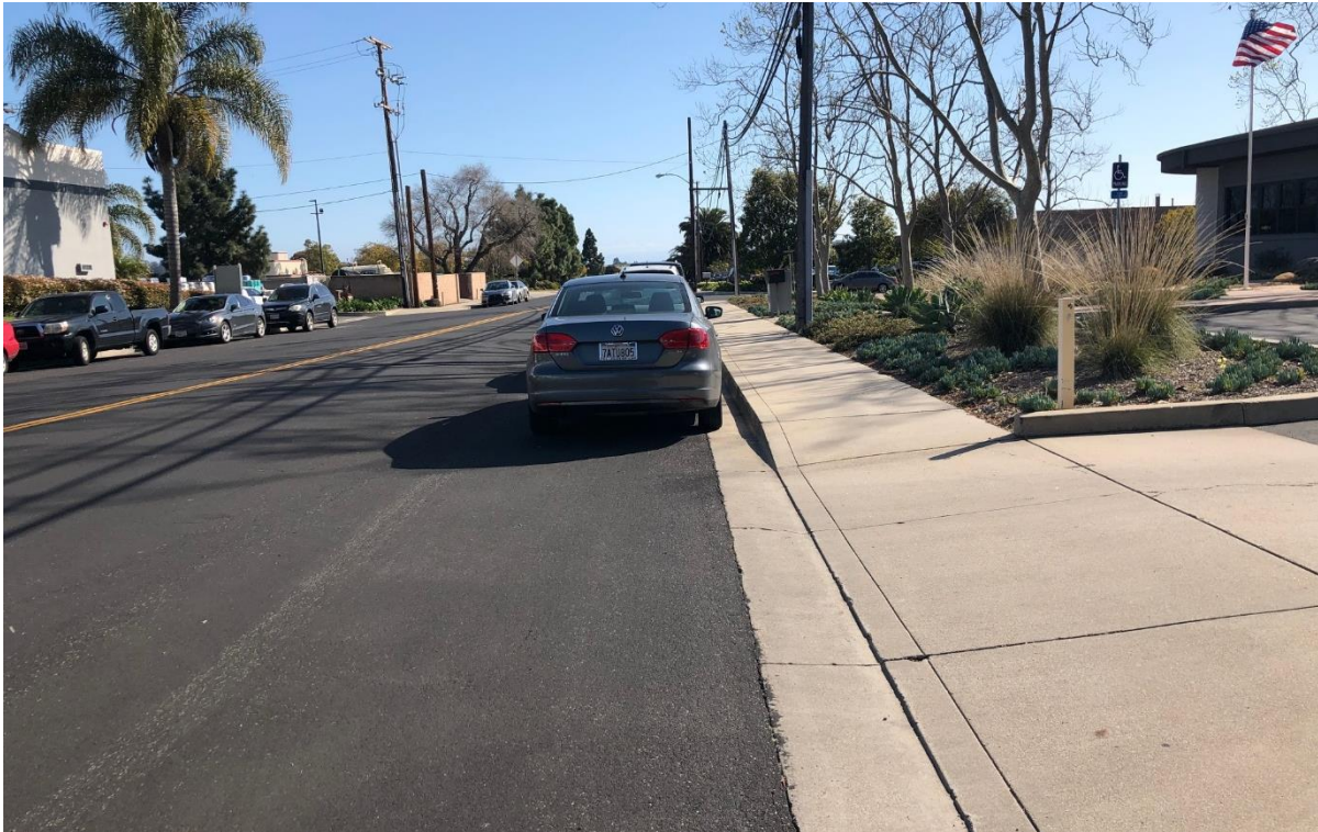
Photograph 1. South La Patera Lane Looking South – With Sidewalk
