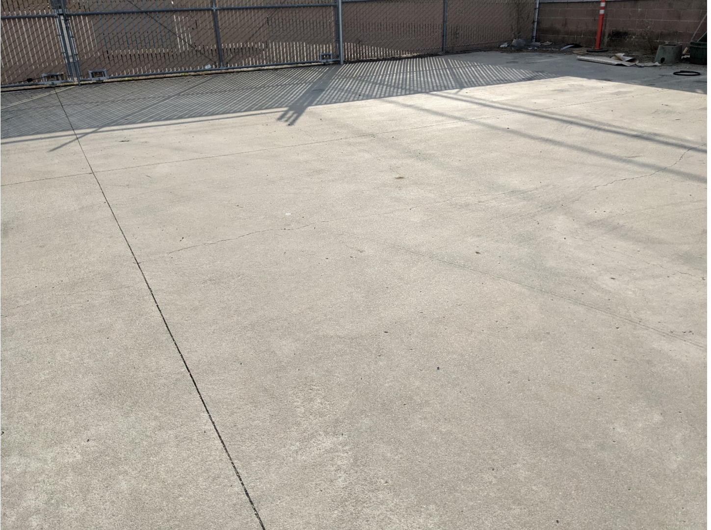
Image 5 – Typical Control Joints
