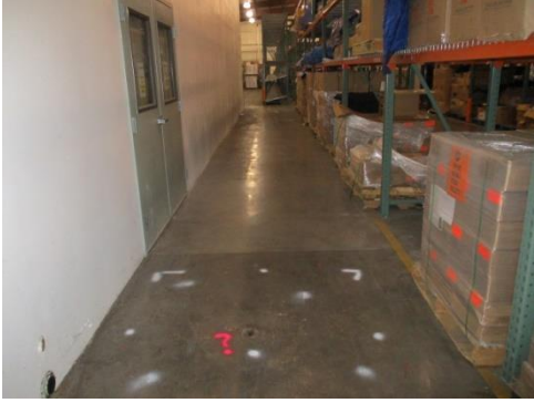
GPR investigation of floor drain in main warehouse.
