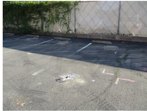
Boring B2 looking south.
