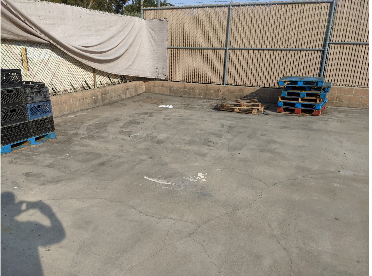
Image 4 – Area Drain at Northwest Corner
