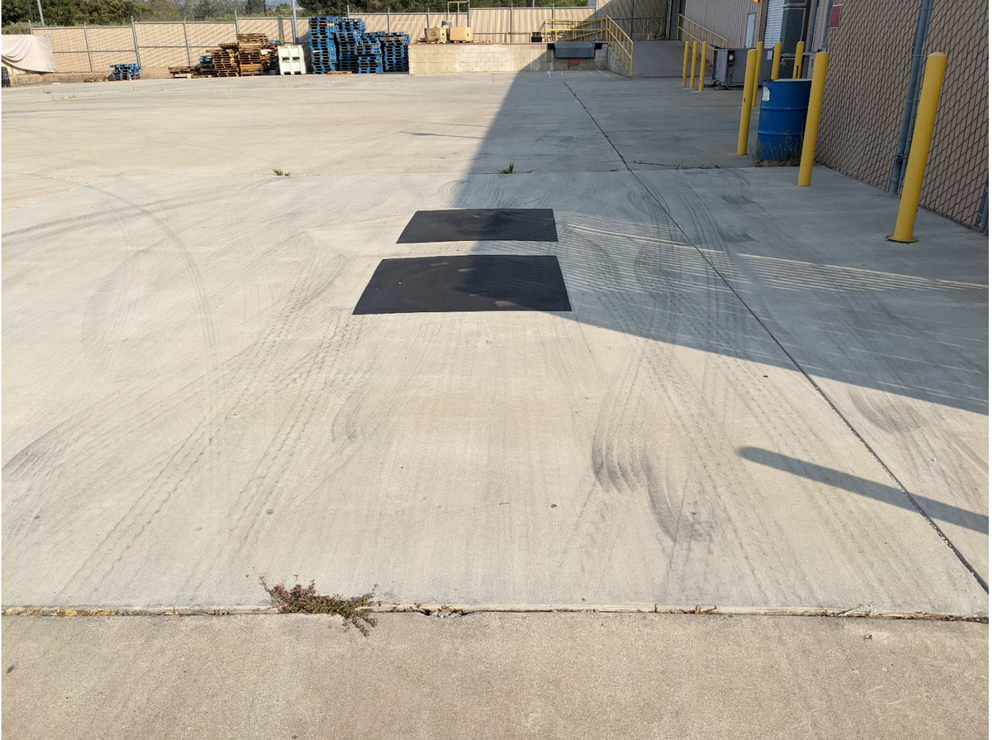
Image 2 – Underground Fuel Tank and Fill Location
