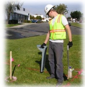
Utility location using the RD4000
