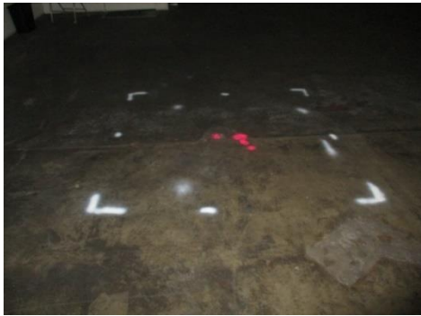
GPR investigation of pipes in the floor in the southeast corner of the west warehouse space.
