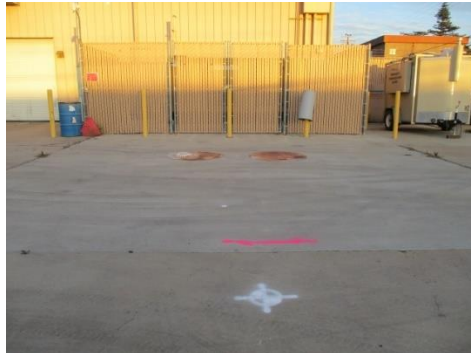
1,800 gallon diesel UST.
