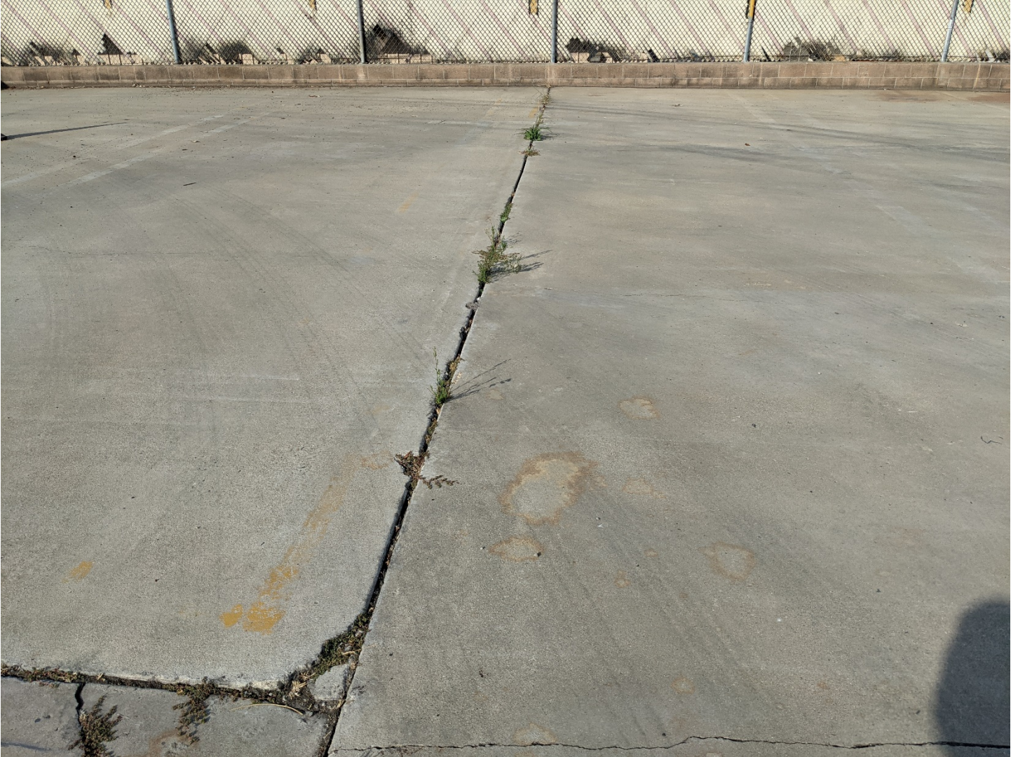
Image 6 – Typical Construction Joint
