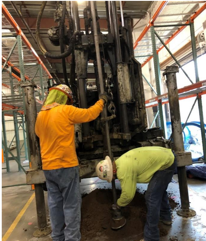
PHOTO 2.3.2-1: Boring Inside Existing Warehouse
