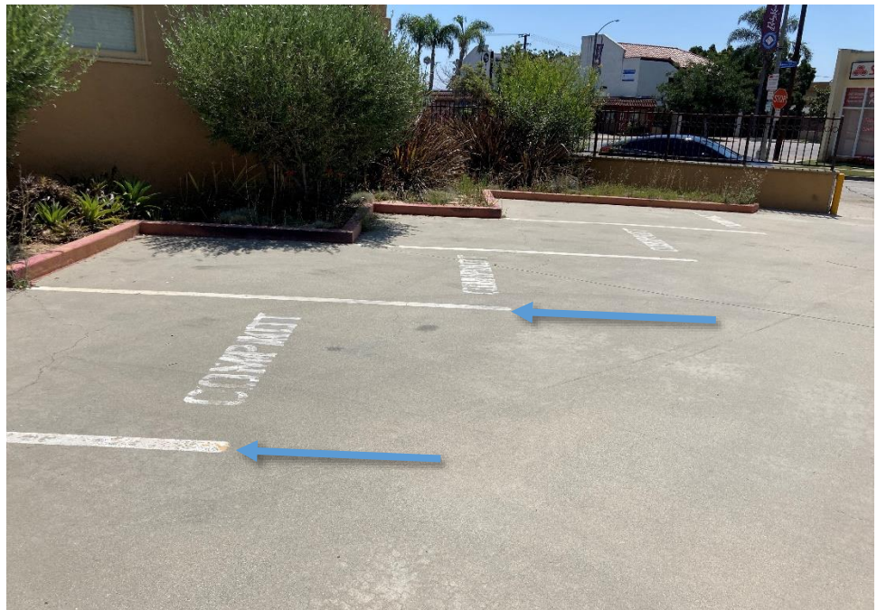
Photograph 6: View of the lead containing white paint in the parking-lot.
