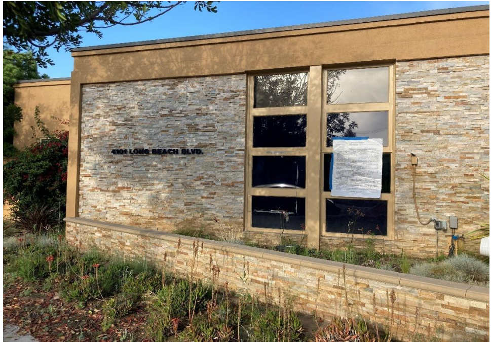
Photograph 1: View of the building located at 4101 Long Beach Boulevard.
