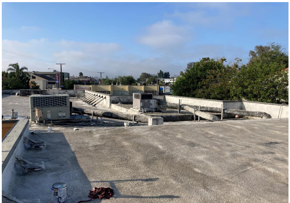
Photograph 2: General view of the roof.
